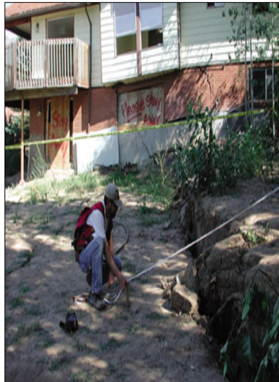
Heather Drive Landslide, Layton (Source: American Geological Institute)
